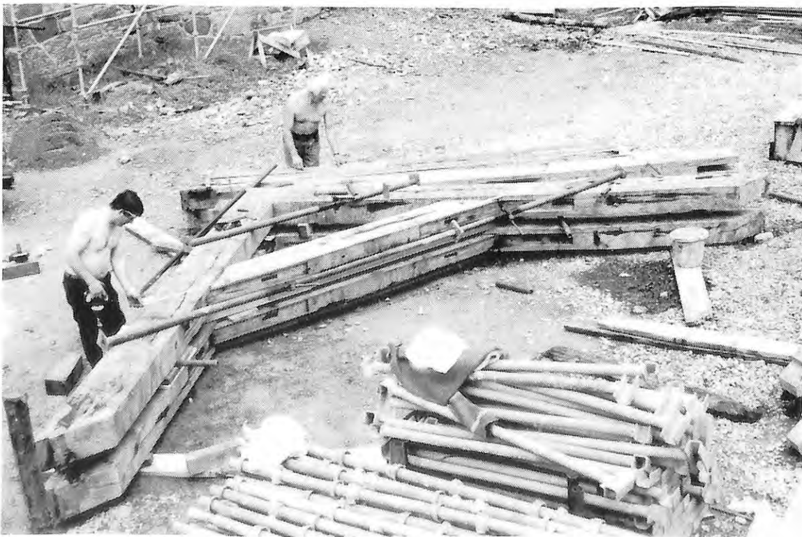
Preparing the roof timbers for Donegal Castle.
