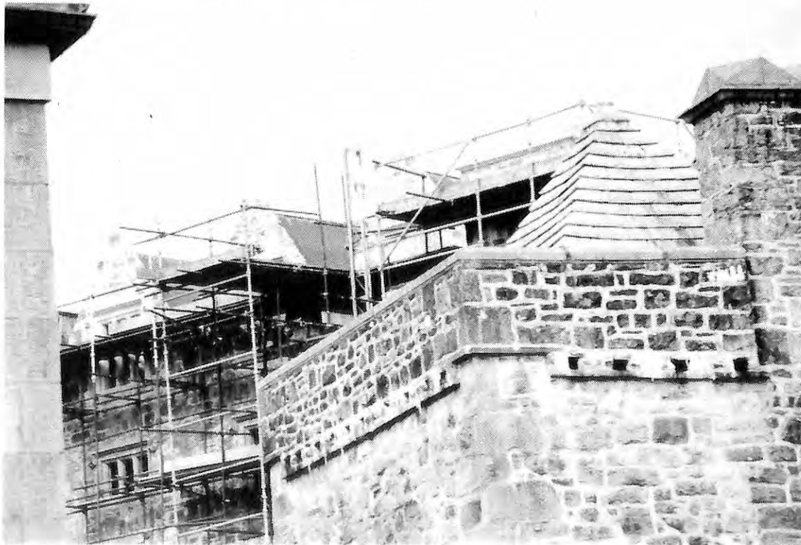
Re-roofing of Donegal Castle still in progress.
